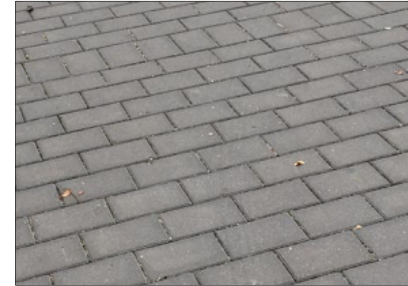
1: Decorative concrete pavers
